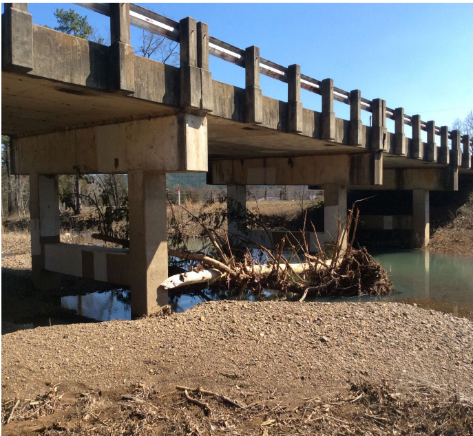
PHOTO 1 Description Span # 3 drift accumulation.
