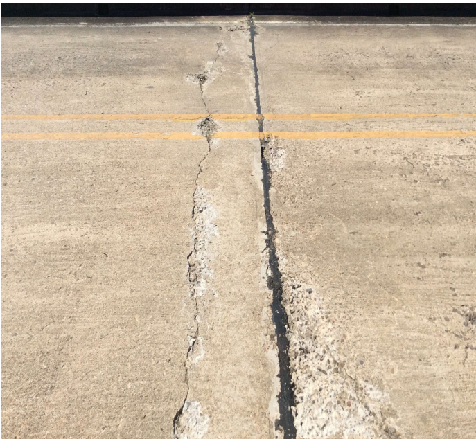
PHOTO 1 Description The deck joint sealant is deteriorating, leaks water and has a few minor areas where the seal is completely missing.
